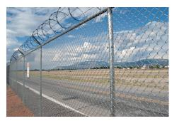
GAW fabric, also referred to as *Galvanized After Weaving*, provides exceptional security and protection. Produced from wire which is first woven into fabric and then galvanized with a zinc coating, GAW is the only chain link fabric that is coated after weaving, ensuring that all surfaces of the base metal are protected against rust and corrosion.
